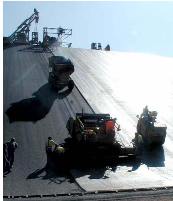
Picture 1.1: Winder (ahead), feeder (middle) and paver and roll (below) at paving a water support basin
