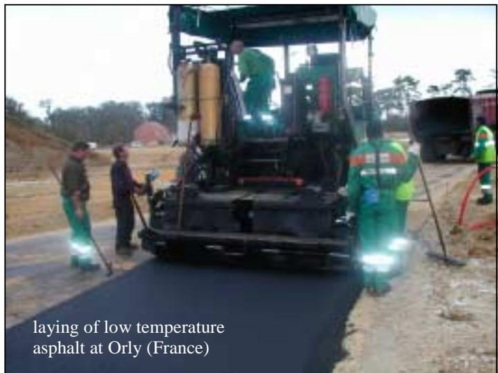
laying of low temperature asphalt at Orly (France)
