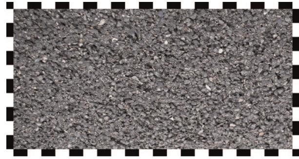
Figure 3. Photograph of the LOA 5 D surface layer in Mecumstraße in Düsseldorf after 30 months of service. The area of the photographed surface is 20 by 10 cm in size.
