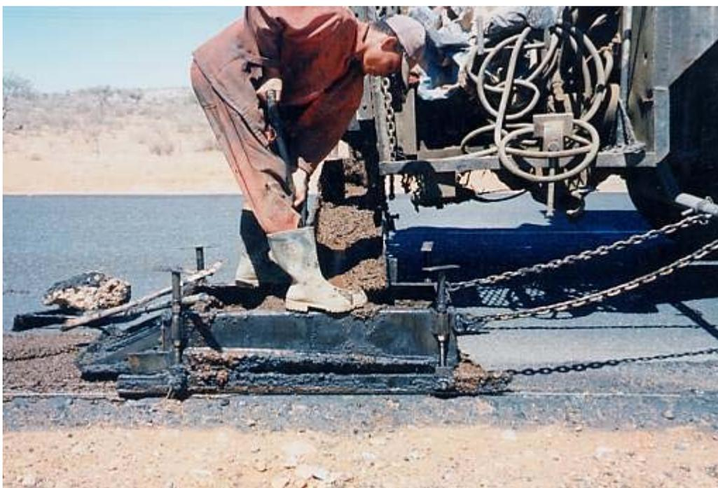
Picture 2. Placing coarse graded slurry.
