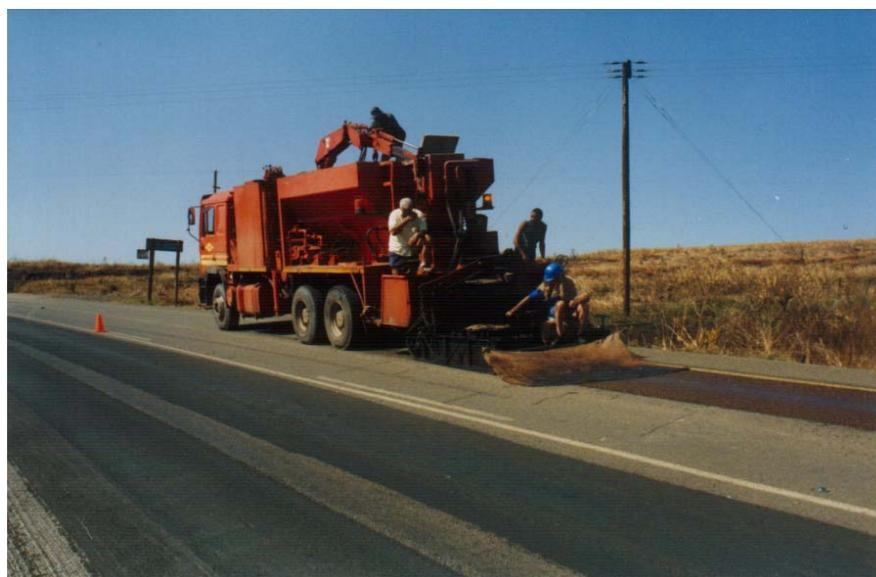
Figure 6. Rutfilling on P22/2 Ixopo to Highflats.
