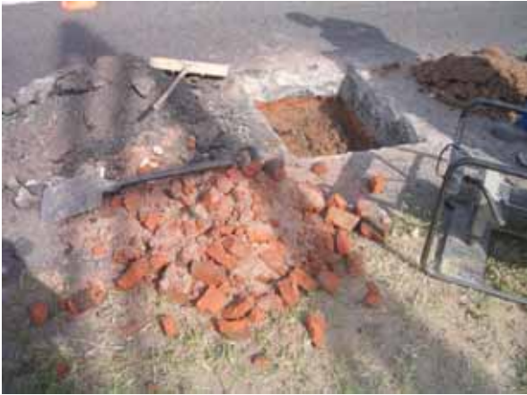
HIGGINSON HIGHWAY REHABILITATION INVESTIGATION JUNE 2010
