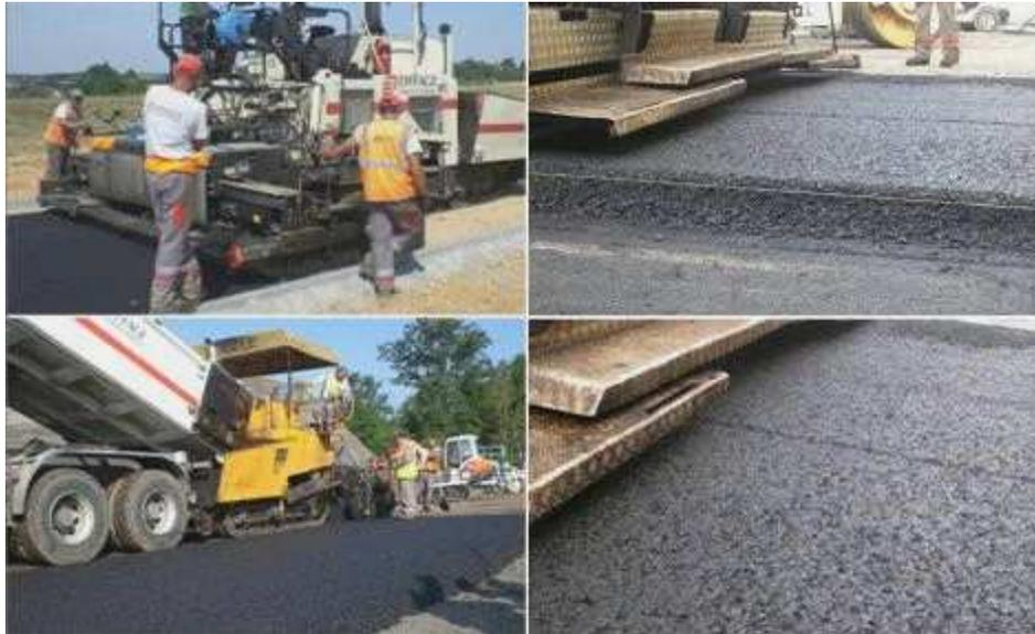
Figure 8 – Paving GB5<sup>®</sup> 0/14mm high-performance asphalt with Noubleau aggregates and 35/45B bitumen in the Tours area. In-place density: 96.4% ; stiffness modulus measured in indirect tension configuration  $E^*(15^\circ\text{C}-10\text{Hz})$ : 14,100MPa.
