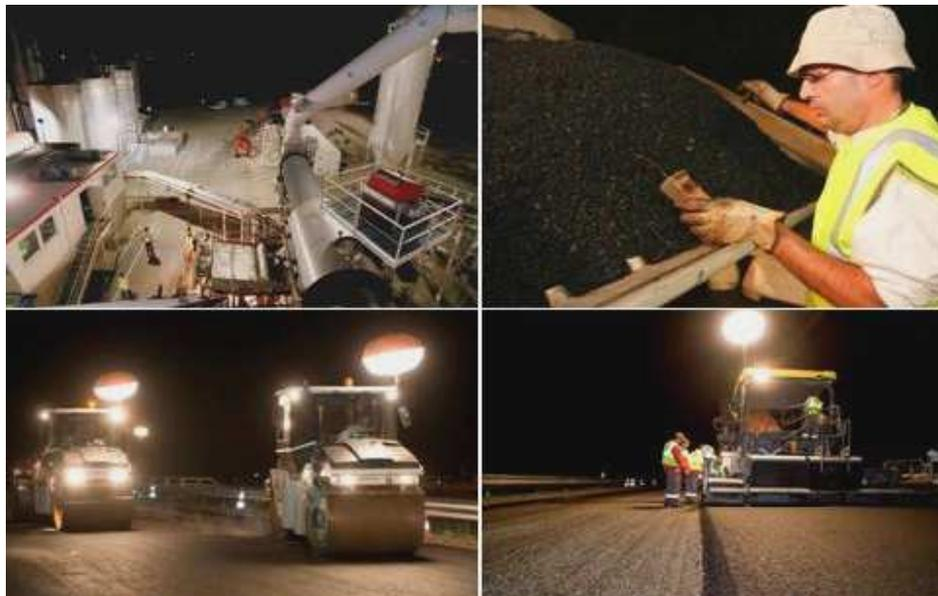
Figure 9 – Paving GB5<sup>®</sup> 0/14mm high-performance asphalt with Cemex aggregates and 35/45B bitumen and 35% RAP (reclaimed asphalt pavement) near Toulouse. In-place density: 97% ; stiffness modulus in indirect tension mode  $E^*(15^\circ\text{C}-10\text{Hz})$ : 15,100MPa.
