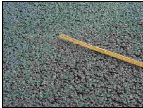
Figure 1: Typical UTFC Surface Texture
