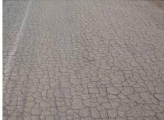
**Photograph 1 Surfacing cracking**
