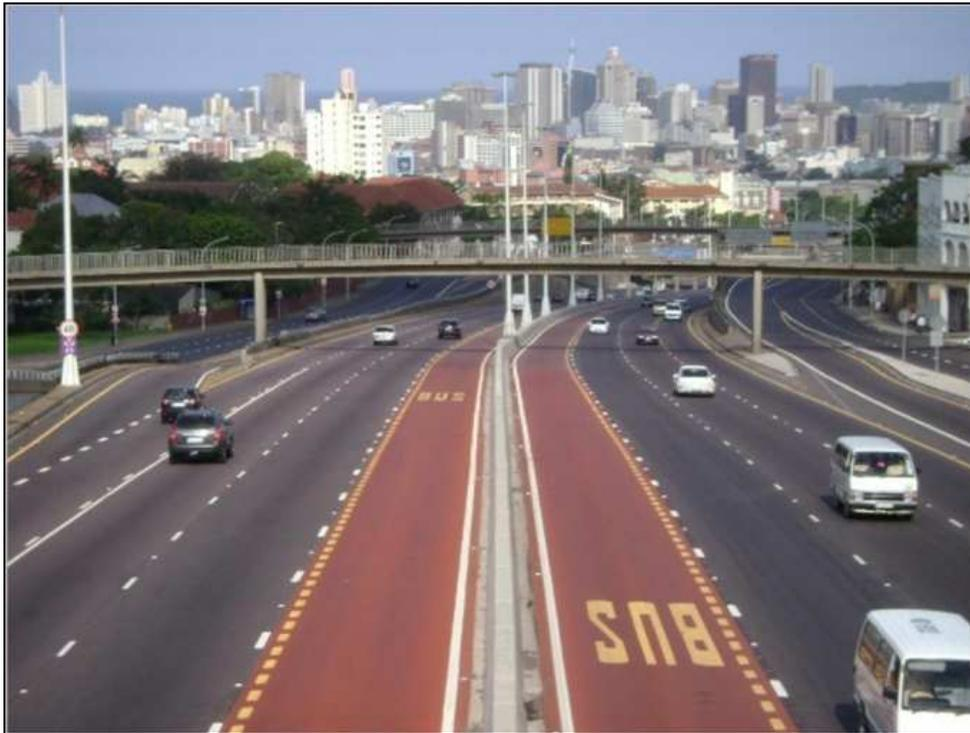
Figure 1: Red continuously graded colourless binder Asphalt on Durban BRT Route<sup>2</sup>
