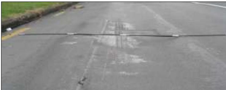
Figure 9: This picture shows rutting/shoving and an unstable asphalt surfacing in a high stress braking area. An investigation was undertaken to confirm causes.
