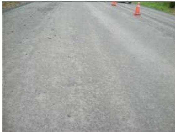
Figure 14: Exposed FBS basecourse prior to reseal
