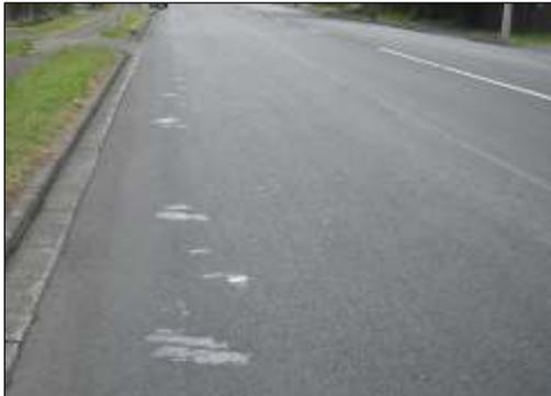
Figure 7: Membrane seal ‘bleeding’ through thin asphalt surfacing. Note line of ‘blooms’
