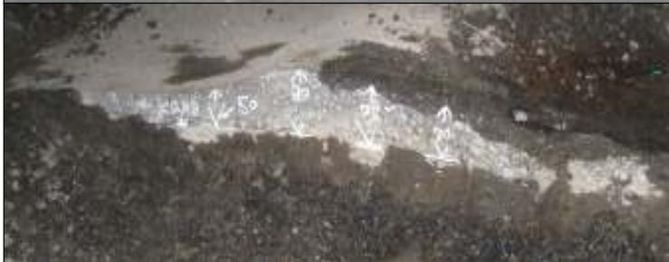
Figure 10: Trenching by the Client confirmed relief was entirely in membrane / asphalt surfacing with a level FBR surface
