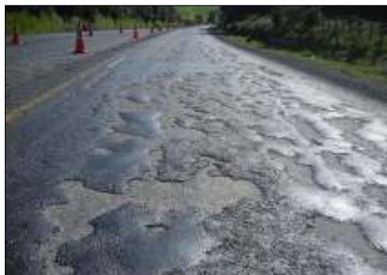
Figure 12: October '07 major surfacing failure
