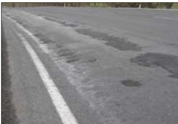
Figure 11: June '07 Primary wheel track repairs
