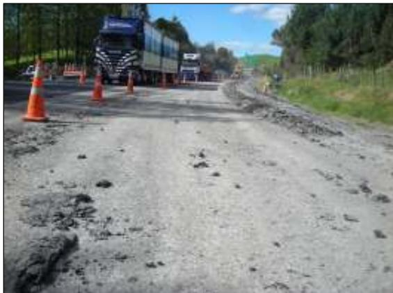
Figure 13: Removal of all seal
