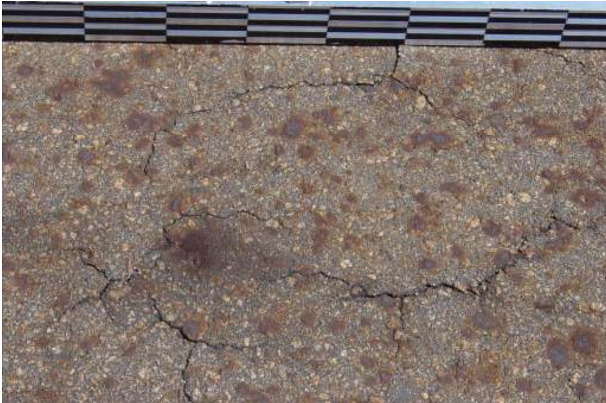
**Figure 1. Typical Cracking and Staining (scale in 100 mm intervals)**
