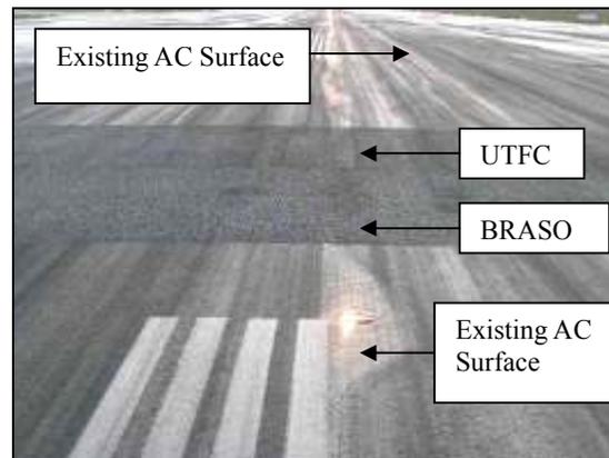
Figure 2.2 Water Run-Off Illustrations Comparison with Existing AC Surfacing
