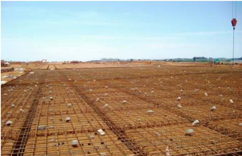
**Figure 5: Concrete raft foundation reinforcement**
