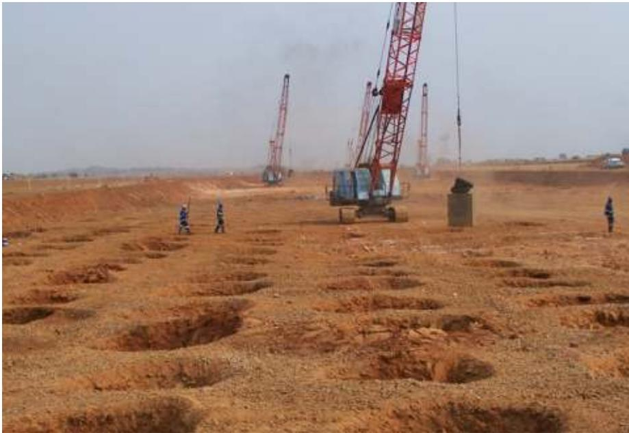
Figure 4: Dynamic Compaction in progress
