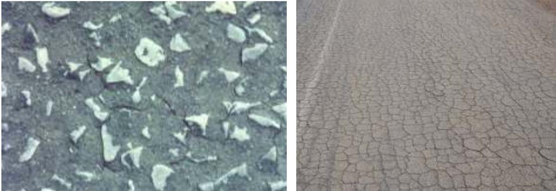
**Photograph 1 Surfacing cracking**
