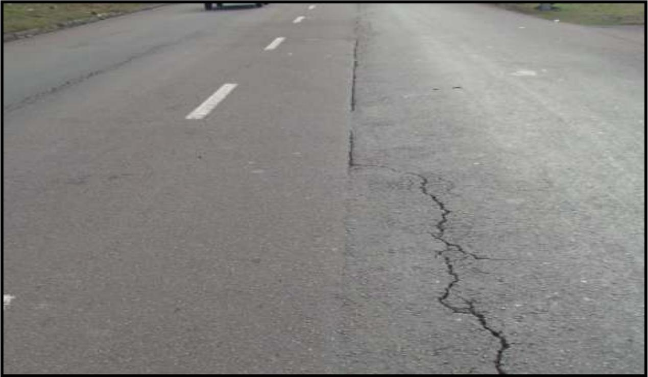
Figure 3: Longitudinal cracks on Bayhead Road
