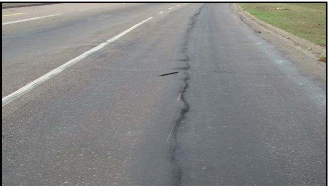
Figure 4: Depression on the asphalt layer on Bayhead Road
