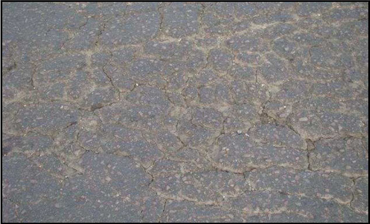
Figure 2: Crocodile cracks on Maydon Road
