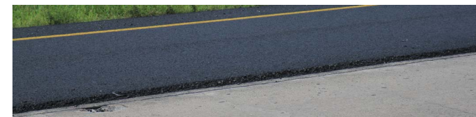
Virginia DoT - Warm Mix SMA on cracked concrete pavement
